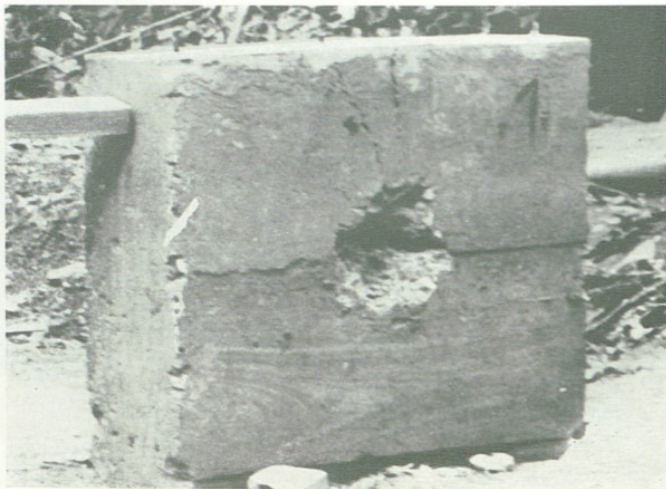
Masonry demolished by grenade fire
